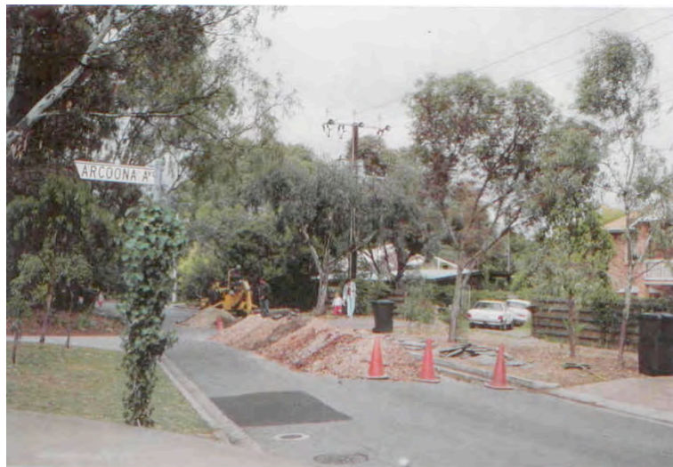
Figure 2.2: Trenching starts April 1990
