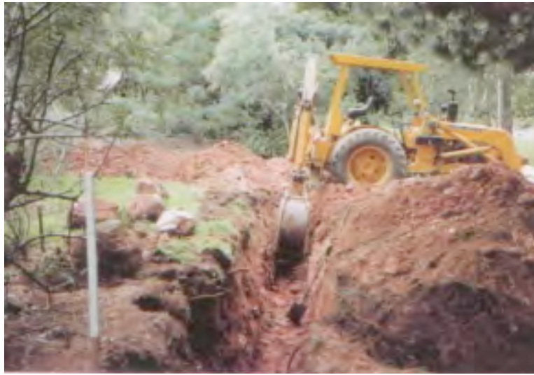
Figure 2.3: Trench digger June 1990
